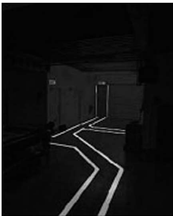
Figure 52: A 'way-guidance' system
